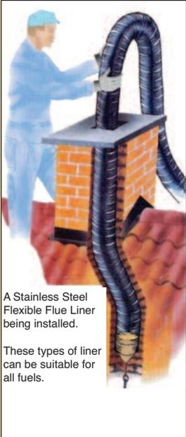
A Stainless Steel Flexible Flue Liner being installed.
